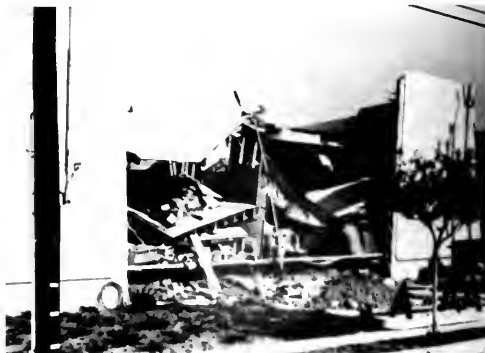
Photo 15. Tilt-up wall panel failed, bringing down portions of the roof and mezzanine floor. Arroyo light industrial tract. See also photo 16. John Meehon photo.
